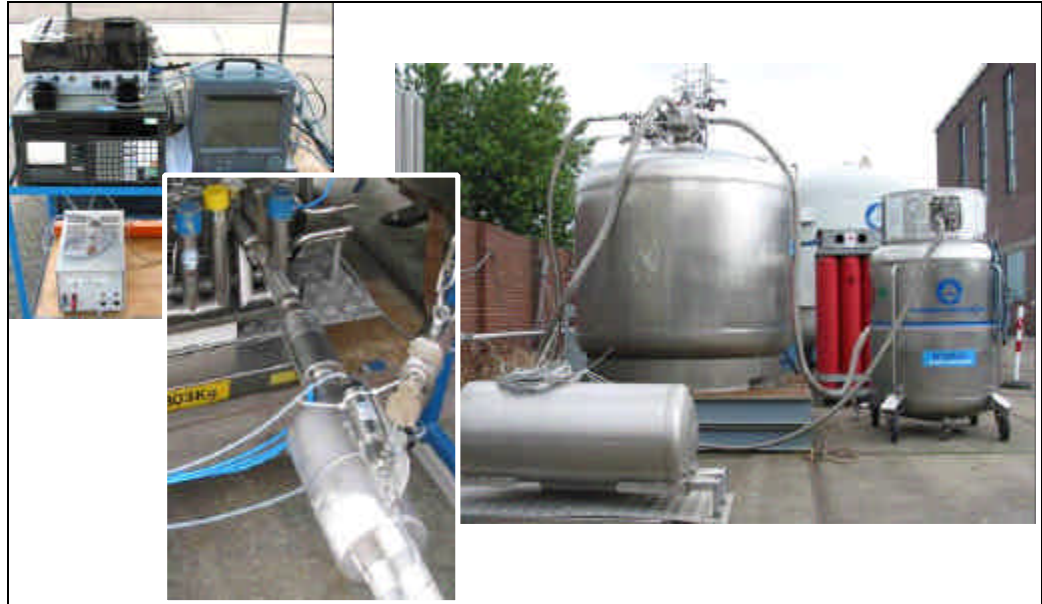
Fig. 5: Equipment for Test Fuelling of LH2 Storage Tank
